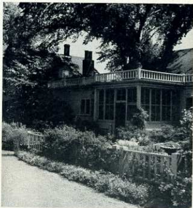
View of side of house with corner of dooryard garden.
